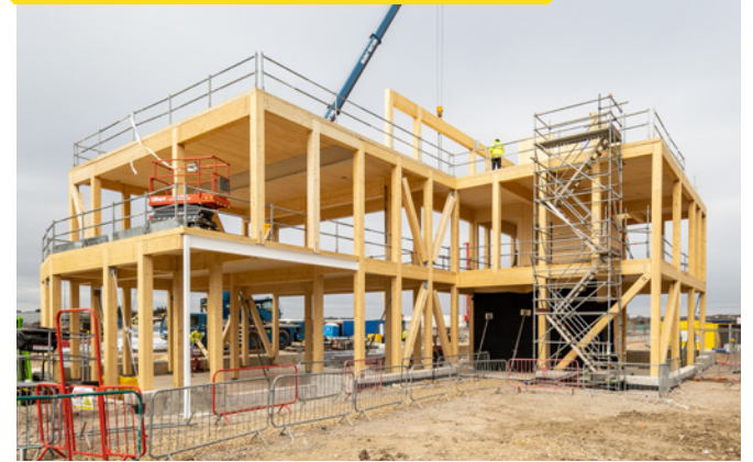
Visitor Pavilion Cross laminated timber frame
